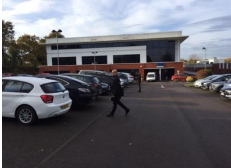
A modern industrial and office HQ facility comprising 129,770 sq. ft. let to Ricardo PLC.
